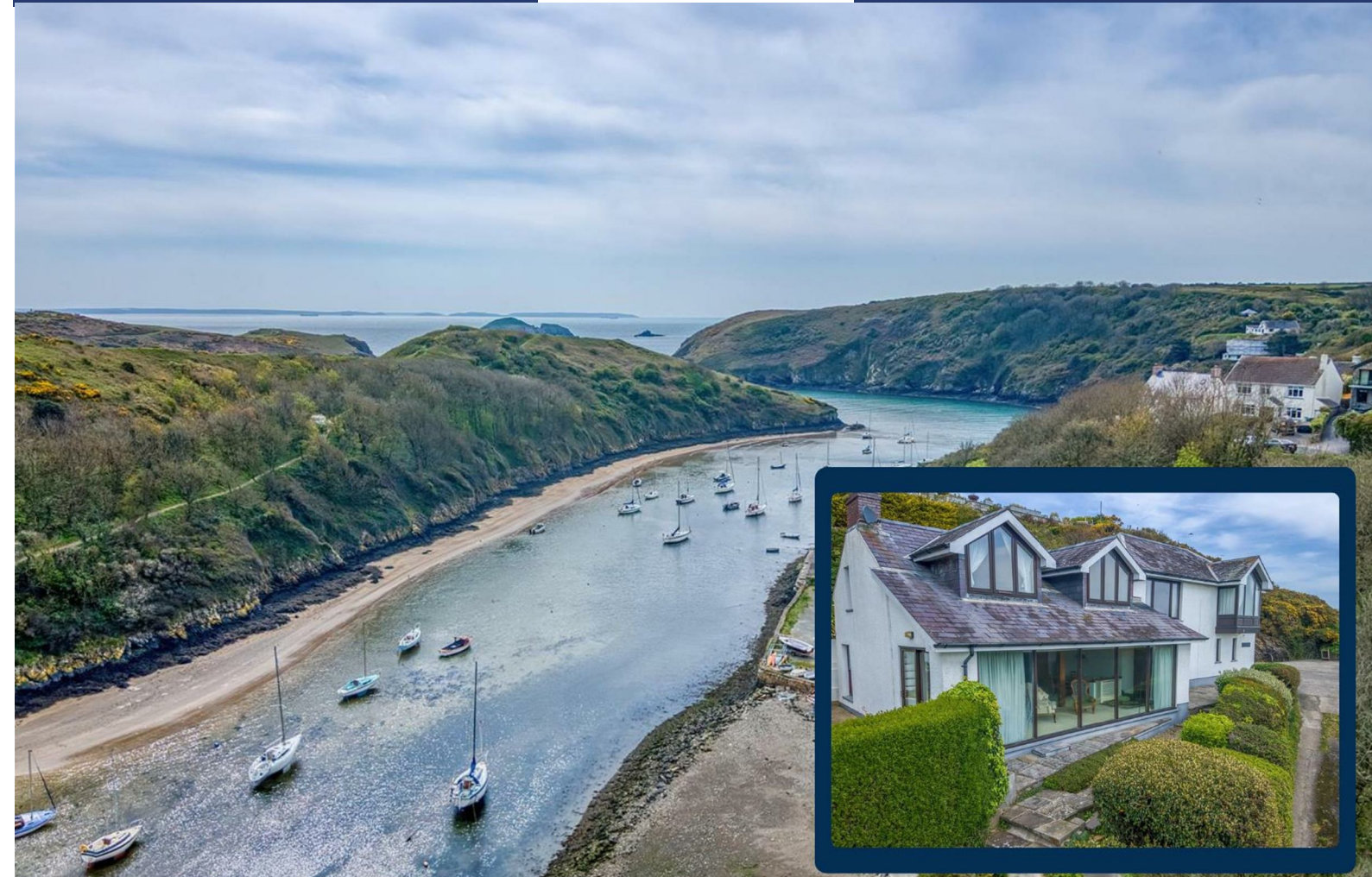
Quarry Cottage The Quick, Solva, Haverfordwest, SA62 6UP
